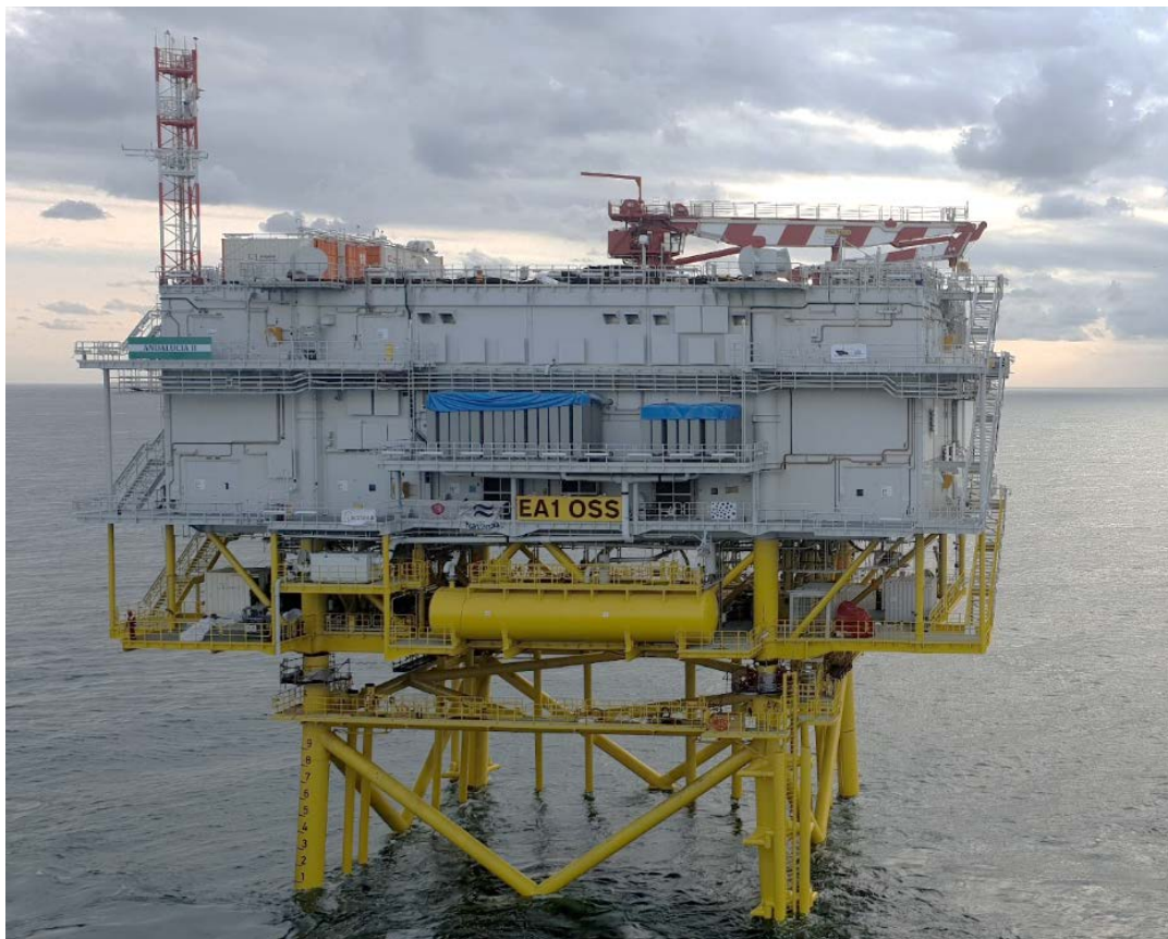
Plate 2.4 Offshore Electrical Platform
